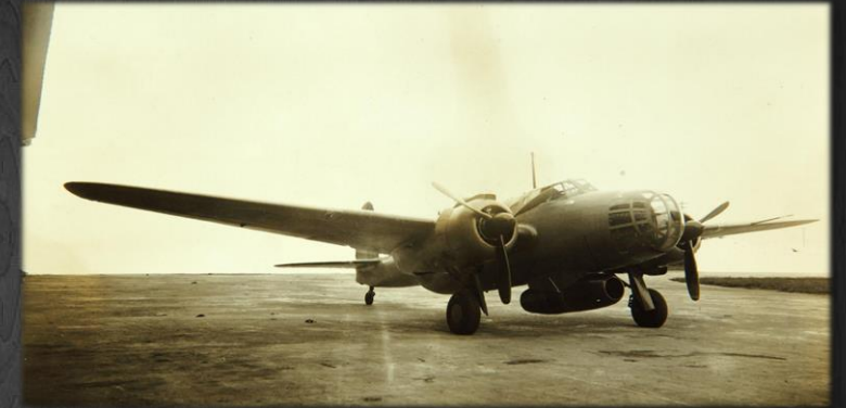
A Kawasaki Ki-48 Lily with a turbojet modification mounted under the main fuselage. This prototype did not see combat.
